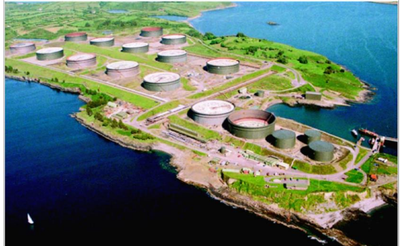
Bantry Bay Oil Storage Facility
